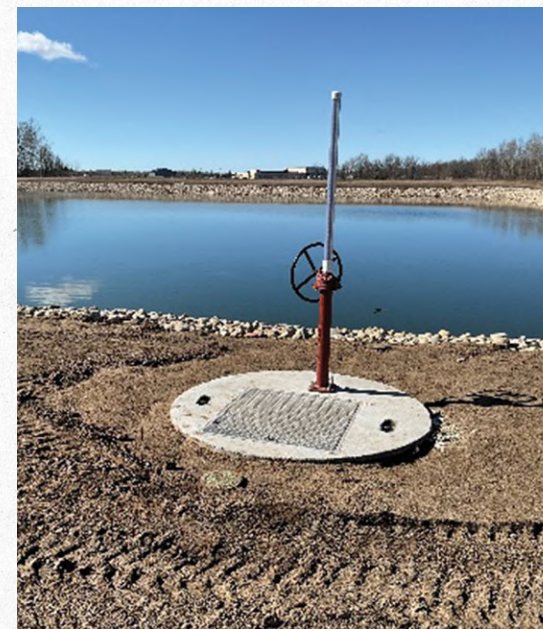
COMPLETED POND CELL PINE POINT WASTEWATER PONDS
