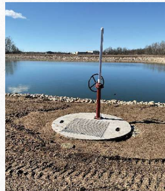
COMPLETED POND CELL PINE POINT WASTEWATER PONDS
